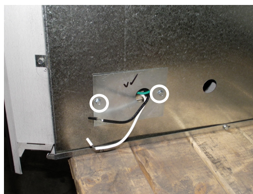
Figure 7 Lead wires that connect to household electrical supply.
