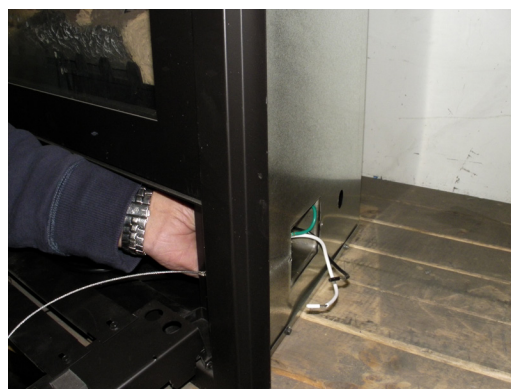
Figure 6 Installing the PPO Box (from outside of fireplace).
